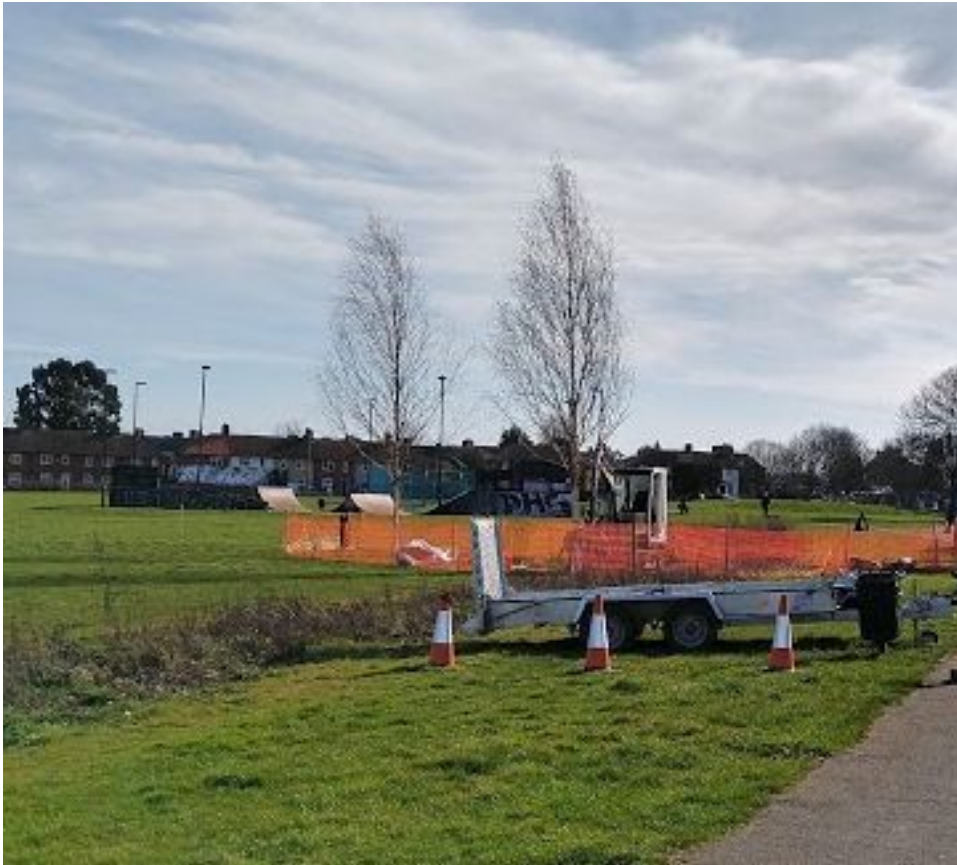
Reflection Garden works underway opposite St Helier Hospital
